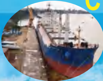
Jetty Service and Berthing Facility
